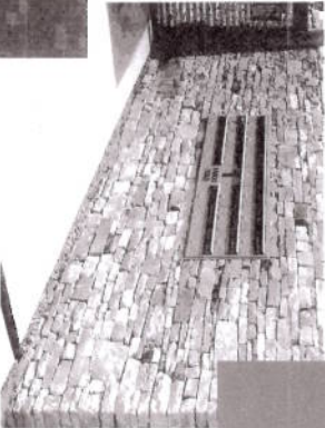
Stone Entry Wall "Drypack Stone"
